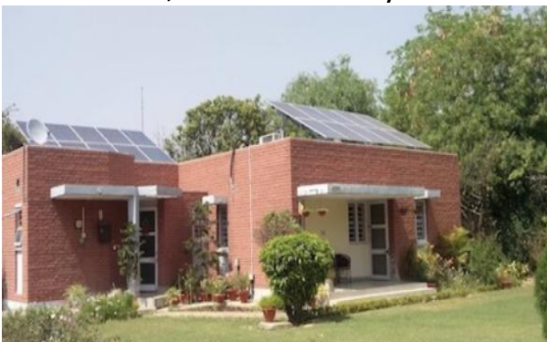
Solar Panel installation at the roof tops
