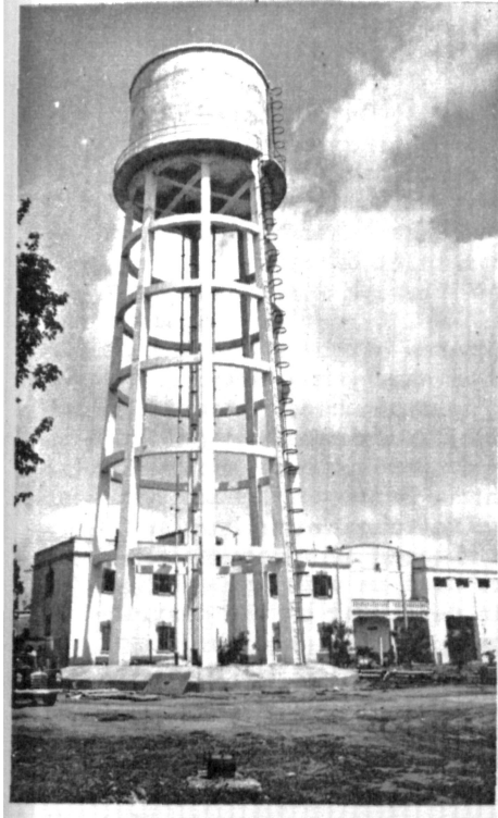
Photo 7 Elevated water tank of reinforced concrete construction near the railway station. No damage of any kind. This is an example of a structure well designed and well constructed following good engineering procedures.
