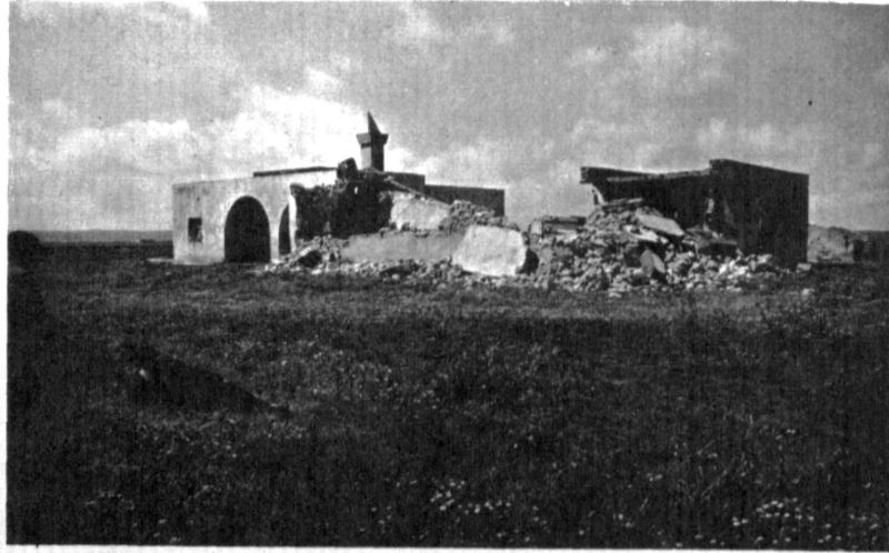
Photo 6 The damage to a wall of hollow concrete block construction of a typical low-cost dwelling house. These housing units are located on the western fringe of the town and they suffered only moderate damage from the recent earthquake. By making certain structural changes in the design and construction, houses of this type of construction may be made adequately earthquake resistant. The low height is an advantage in reducing the weight and seismic stresses. Note the trees in this neighborhood and the happy people. The new site for the reconstructed town of Barce should be located, to save these trees as much as possible.
