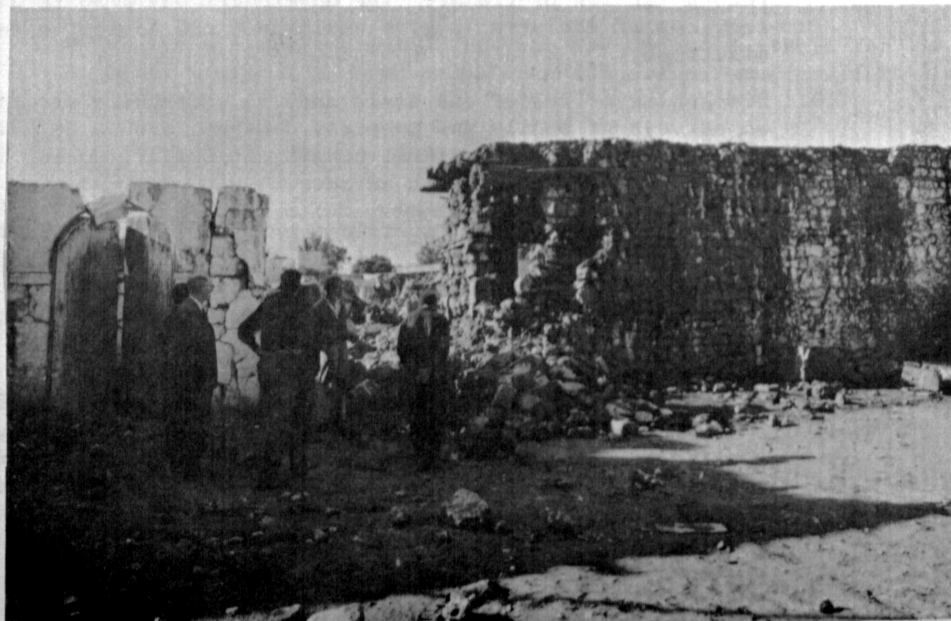
Photo 2 An example of damage to a house of rubble stones embedded in terra rossa. Note the roof construction consisting of stones and mud over wooden rafters.
