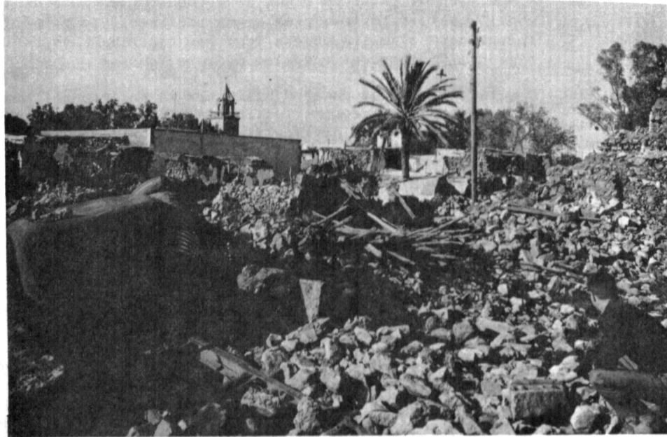
Photo 2 An example of damage to a house of rubble stones embedded in terra rossa. Note the roof construction consisting of stones and mud over wooden rafters.
