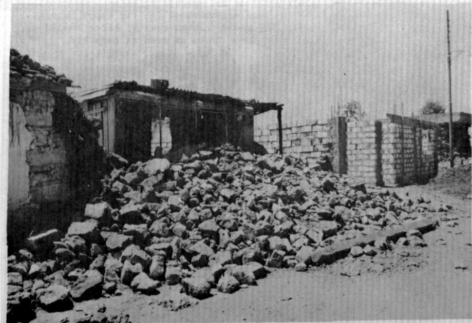
Photo 4 An example of collapse of rubble stone walls which enclosed the inside frame consisting of discarded metallic rolling stock. To the right is a building of stone block under construction which is provided with reinforced concrete columns that was saved from collapse.
