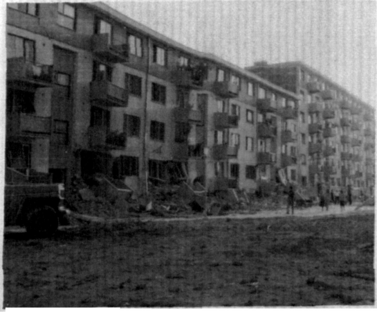
Figure 3-4. Four story brick masonry apartments that collapsed.
