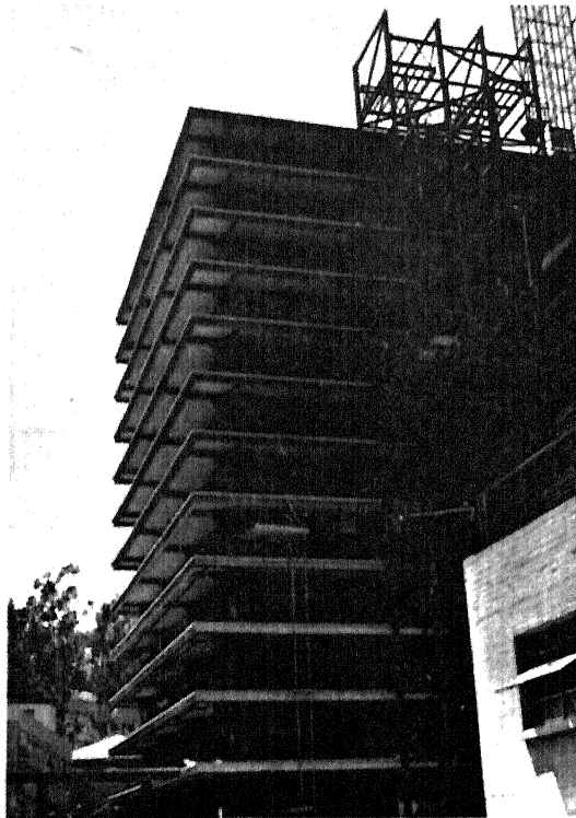
Figure 4. Trussed Frame of East Mechanical Service Tower
