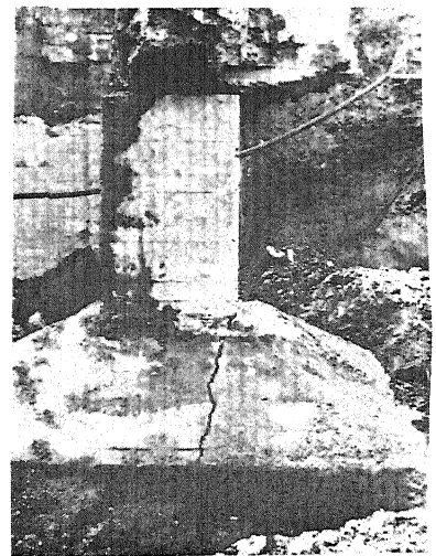
Photo 17. Cracks of the Footing of Interior Column (Hamamatsu Shear Wall Test).
