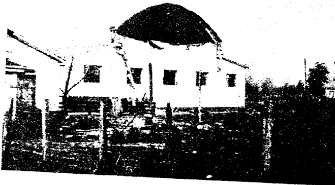
Fig. 1.91 Industrial building near Valdivia. General view.
