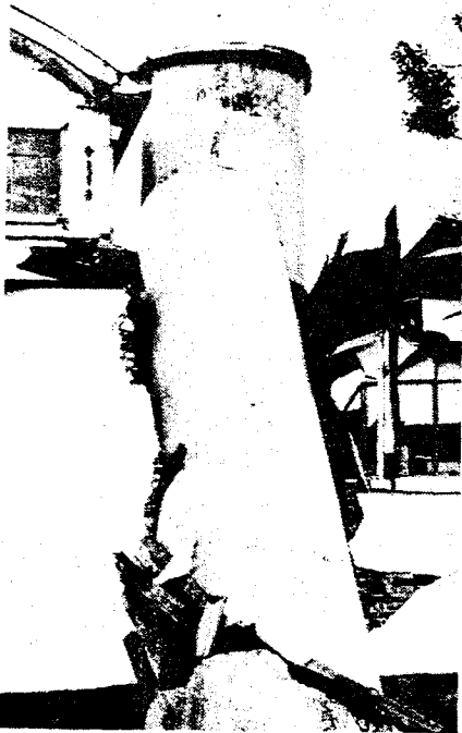
Fig. 1.64 Industrial Plant near Valdivia. Power Plant. Reinforced concrete chimney collapsed at construction joint.
