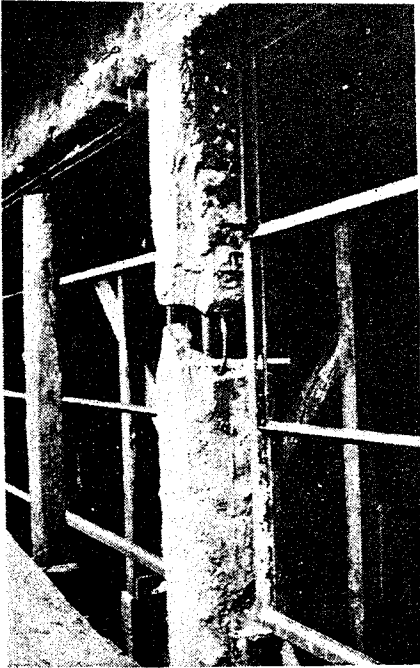
Fig. 1.11 School in Coronel. Two buildings 50 m. long each collided in third floor causing considerable structural damages.
