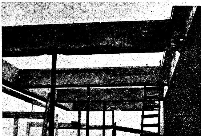
Fig. 1.53 Ditto. Overhanging top structure supported on steel pipe columns.
