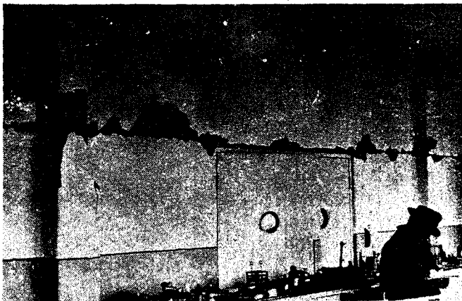
Fig. 2.21 Ditto. Poor bond between masonry and supporting structure.
