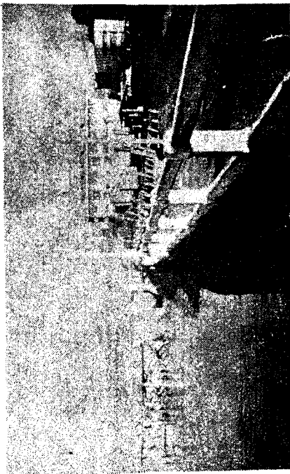
Fig. 1.72 Hotel Puerto Montt. Big sliding on the foundation toward the sea. General view.
