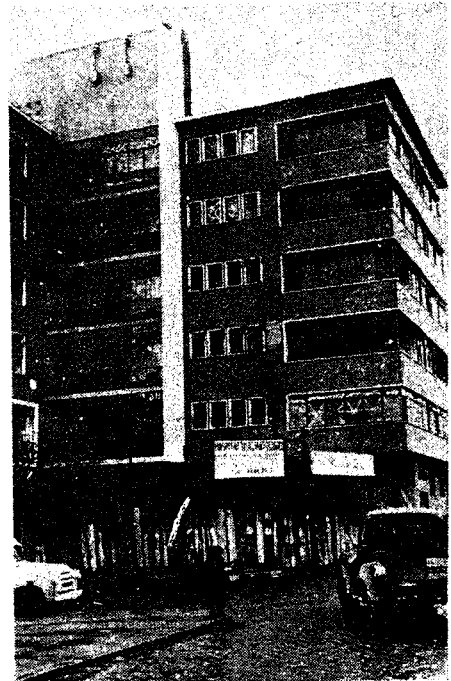
Fig. 1.25 Traumatological Hospital in Valdivia. Highly asymmetric disposition of supporting elements. General view.
