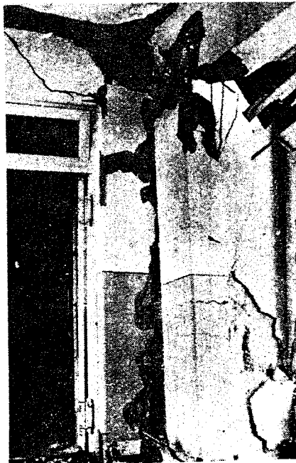
Fig. 1.15 Ditto. Collision between main building and central aisle (7th floor).
