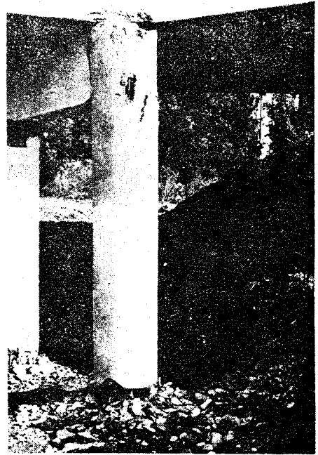
Fig. 1.23 Damage in upper and lower ends of central columns.
