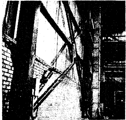
Fig. 15 Mill Buildings - Diagonal Bracing
