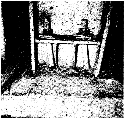
Fig. 16 Mill Buildings - Column Base
