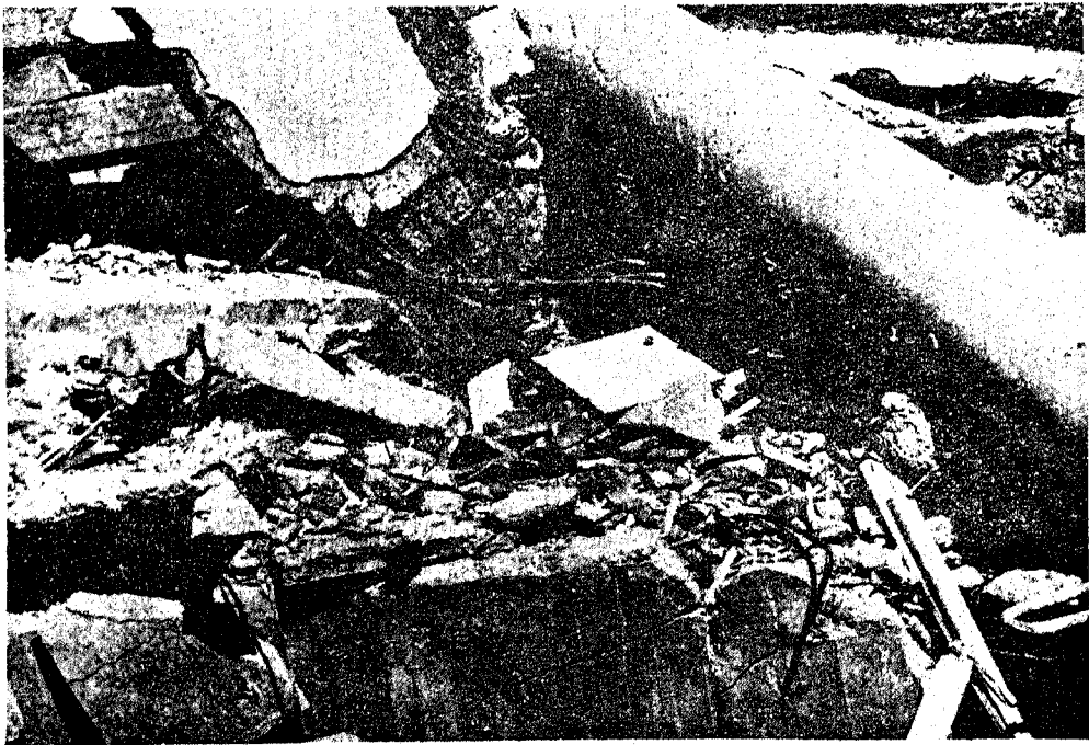
Fig. III-2 Consular Building. Example of defective technical disposals.
