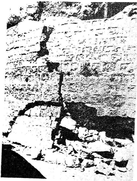
Fig.10.- Forebay basin of the Volcan Plant. The stone wall has failed due to settling of the hill.
