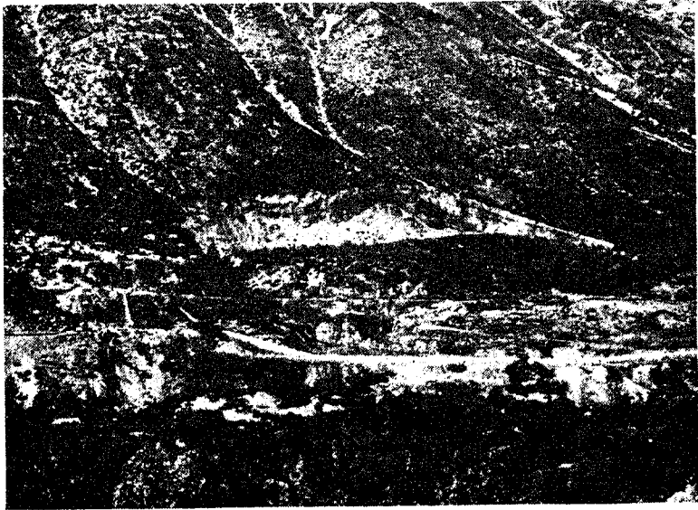
Fig. 4,- Heavy landslide at El Manzanito. A large part of the fracture surface can be observed. Lower down appears the steel siphon that was built to replace the canal.
