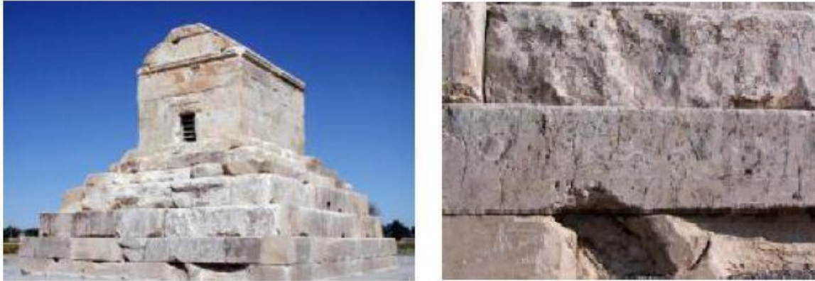
Figure 3. King Cyrus Tomb in Pasargadae (southwest of Iran) built in 550 BC. On the right, a close view of the smoothed cut-stone layers with no mortar between them can be seen.
