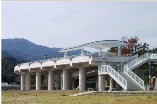
Figure 3. Shirahama tsunami evacuation structure in Japan. Photo by Professor Nobuo Shuto
