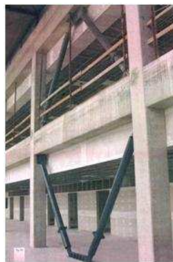
Figure 1. Building protected with BRB
