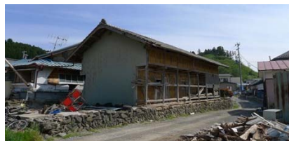
Photo 2.18. Survived soil warehouse which might have comparatively slight structural specifications.
