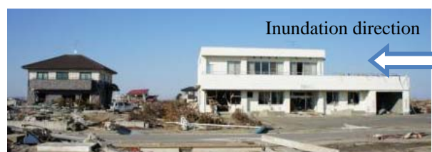
Photo 2.7. Wood house to remain in the downstream of RC building in Arahama, Sendai city.
