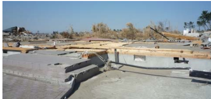
Photo 2.3. Foundations and sills remained.
