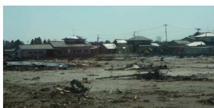
Photo 2.6. Many wood houses remained.
