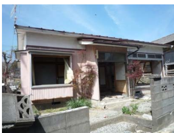
Photo 2.17. Survived house which might have comparatively slight structural specifications.
