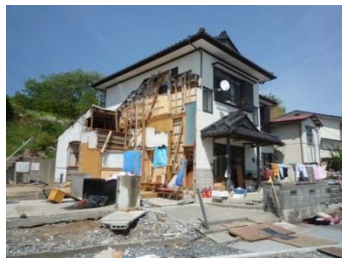
Photo 2.15. Wood house remained under the flood water depth of over 7 m.
