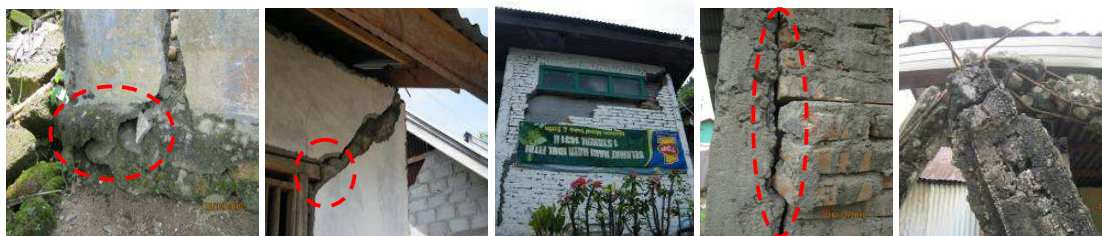
Figure 3: Damage on foundation, corner crack, damage on wall, damage on orthogonal wall & damage on beam column connection (left to right)
