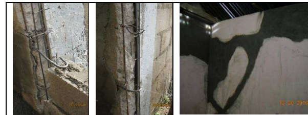
Figure 13: Improper methods: jacketing (left and middle) & crack repairing (right) procurement and supervision
