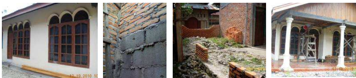
Figure 10: Large opening, different wall materials, no tie beam & pre-cast column (left to right)
