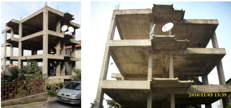
Figure 7. General view of the 1 st Case Study structure
