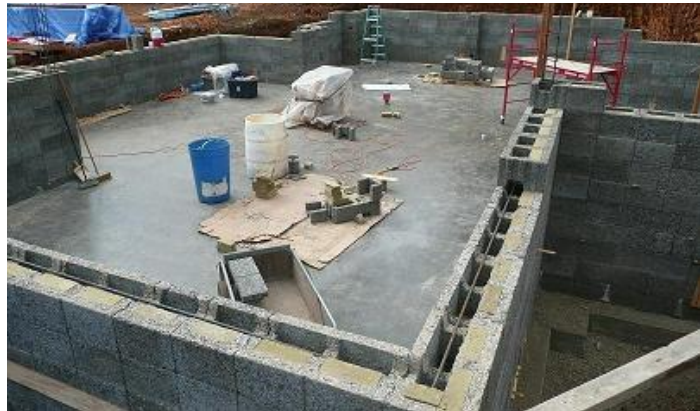
c) Dry-stacking forms into walls (Block B show)
