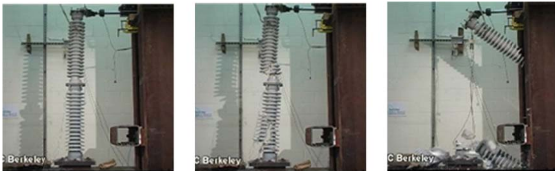
Figure 2.4 Propagation of damage and failure mode of 230-kV porcelain insulator post in fragility test.
