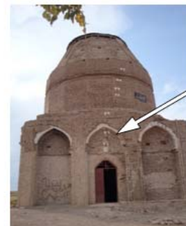
Figure 12. Stresses contour S1 earthquake in direction Y Figure 13. A crack at the top of the arch of the door
