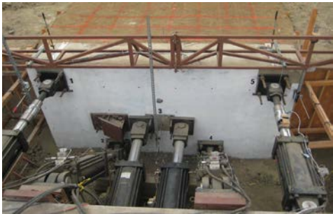
Figure 2.4. Photograph of loading system in the field
