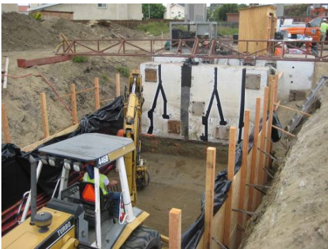
Figure 2.1. Photograph of backwall specimen during construction
