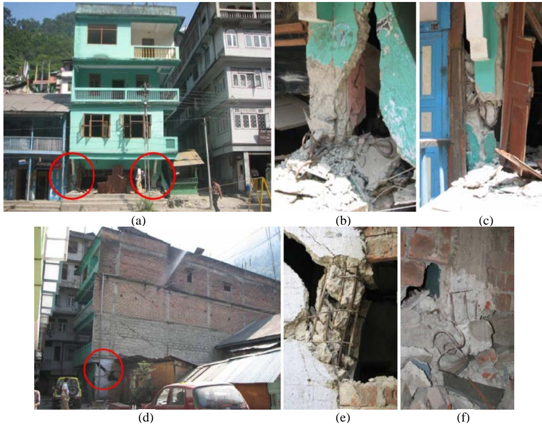
Figure 9. Partial collapse of a four storey RC building at Singtam market during 2011 shaking: (a) Overview of the building with failure of front RC columns, (b), (c) closer views of complete failure of front RC columns, (d) tilting of the building along its length, (e) failure of RC columns on the rear of the building, and (f) failure of an internal RC column showing use of plain reinforcing bars and inadequate provision of shear reinforcement.
