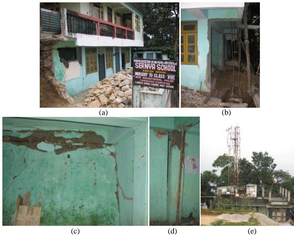
Figure 7. Damage in Sernya School building: (a) partial collapse of portion of first storey, (b) collapse of walls due to ground movement, (c) out-of-plane movement of masonry infill, (d) repair work in first storey, and (e) vibration of mobile communication tower on top of the building damaged the supporting RC column.
