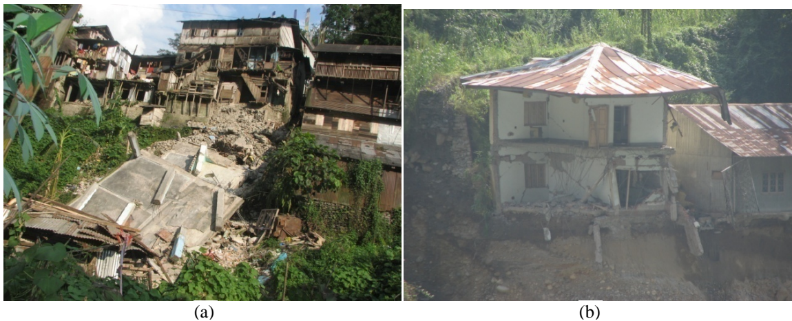
Figure 8. (a) Collapsed four storey RC building at Dikchu bazaar; (b) a part of two storey RC building near Dikchu dam site collapsed during 2011 shaking.
