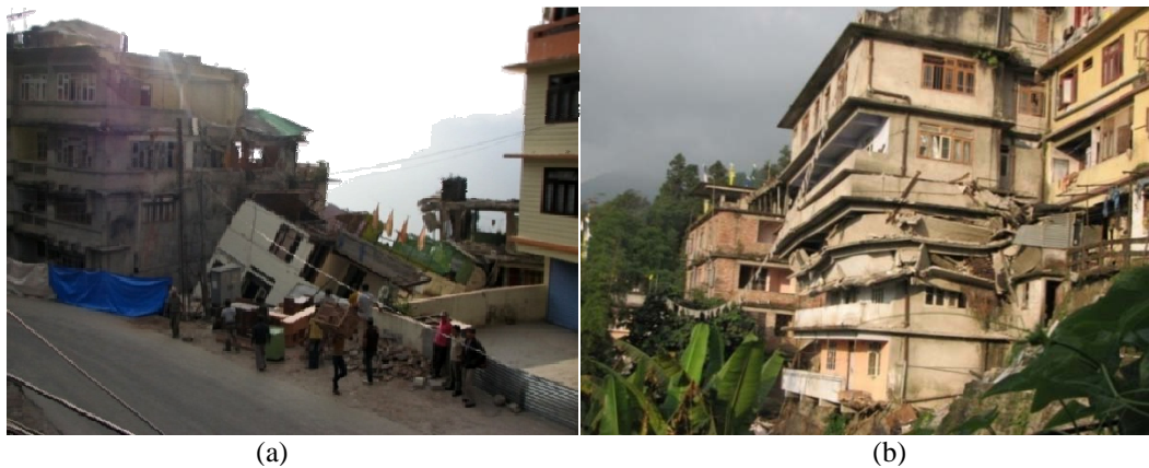
Figure 10. Collapse of two RC buildings at Baluwakhani in Gangtok: (a) the six storey building collapsed completely due to foundation failure, and (b) adjacent nine storey building suffered pan-cake type collapse in intermediate three stories.
