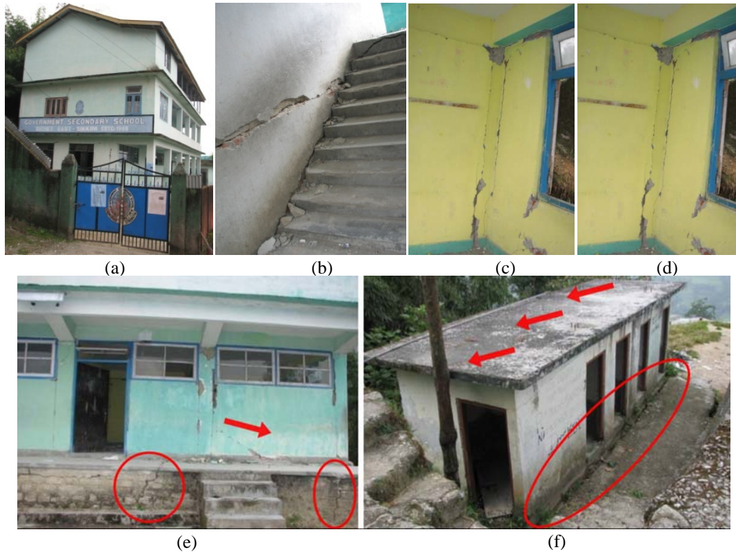
Figure 6. Government Secondary School, Sichey: (a) overview of renovated old school building, (b) damages in staircase, (c) separation of masonry blocks along beam-column interfaces, (d) damage to RC columns, (e) cracks in corridor of new school building, and (f) separation crack in pavement beside toilet block.
