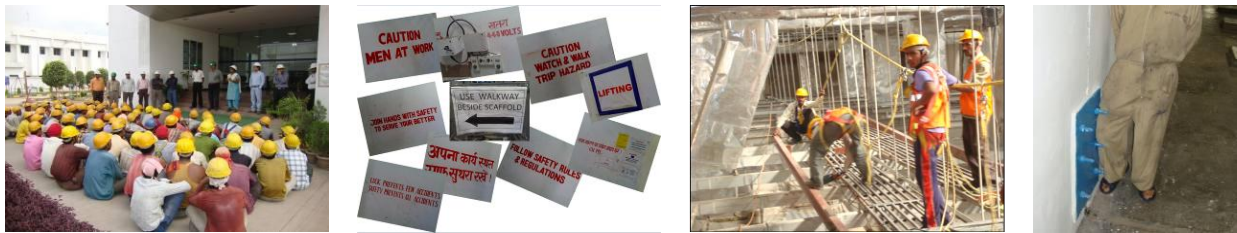
Figure 17. Tool box meetings, multi lingual safety signs, clip on when working at height and hazard identification
