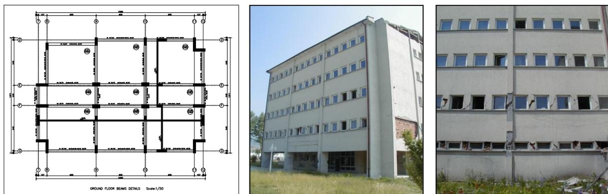
**Figure 4.1.** Ground floor plan and observed damage state after Nov.12, 1999 Düzce Earthquake
