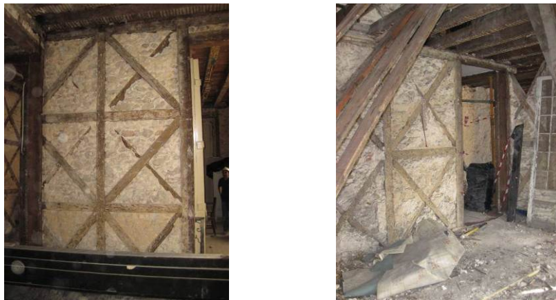
Figure 1. Frontal wall in “pombalino” Building (Gonçalves, et al. 2011)
