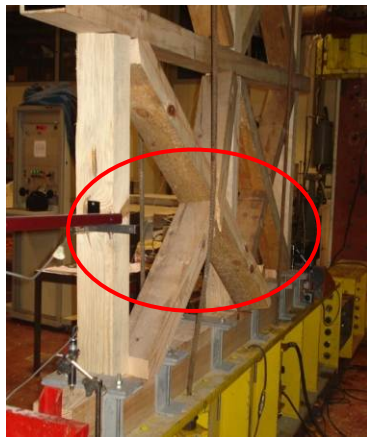
a) Failure by buckling of diagonal for TF1
