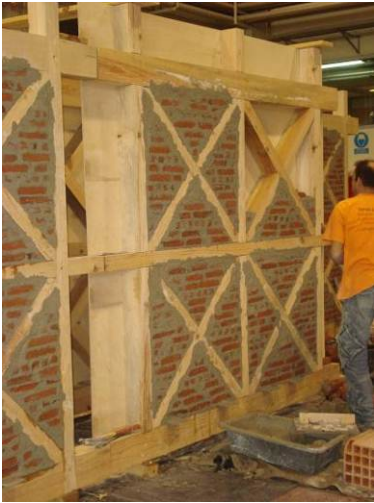
Figure 4. Masonry wall fabrication
