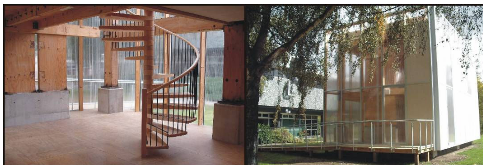
Figure 1.2. The Expan Office Structure for STIC
