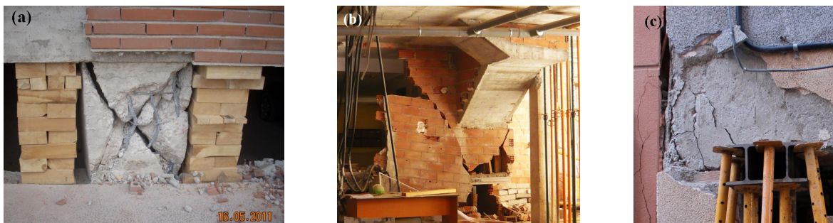
Figure 5. Brittle failures in RC columns; (b) and (c) (Calconsa XXI 2011).
