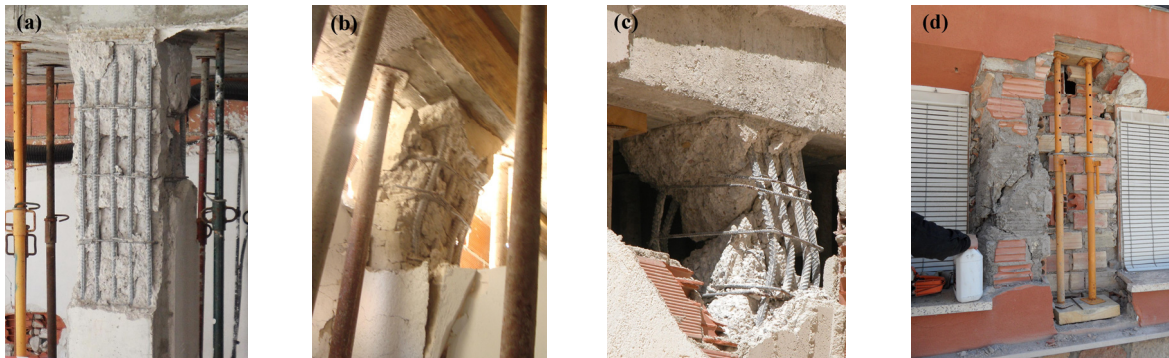
Figure 5. Brittle failures in RC columns; (b) and (c) (Calconsa XXI 2011).
