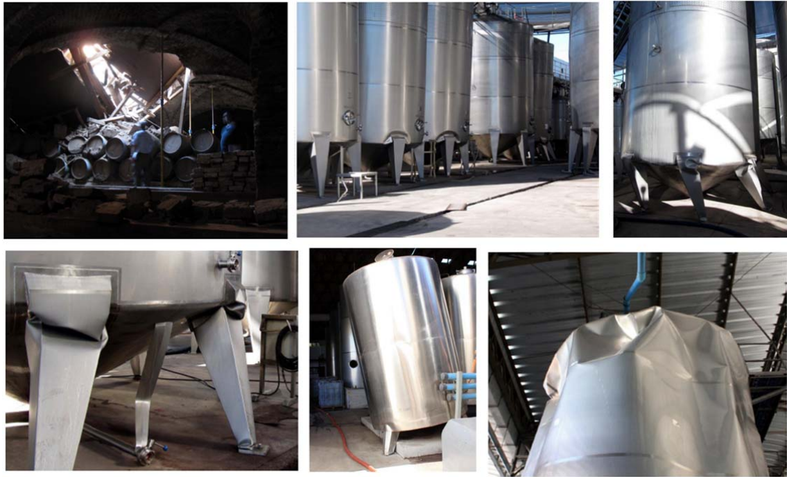
Figure 5.- Damage photos Brewery.
