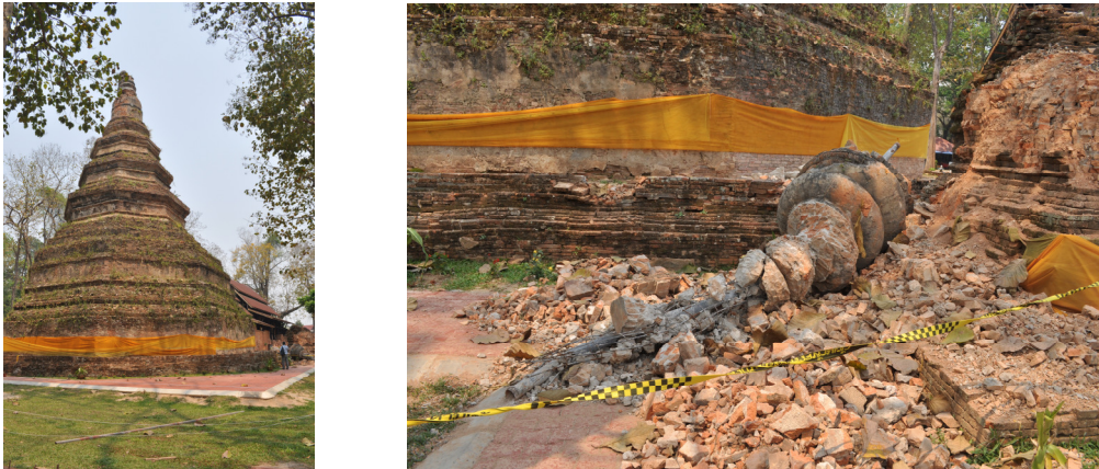
Figure 5. Damage to a pagoda in Chiang-saen District
