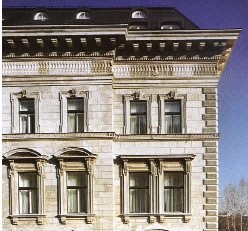
Figure 2. Palais Leitenberger, 1871/1872 with typical façade elements.
