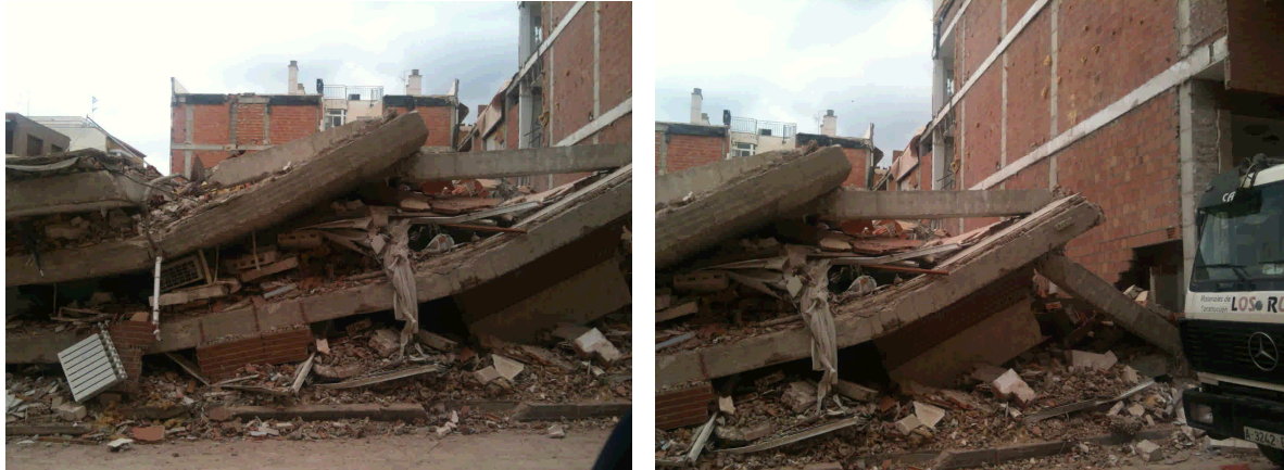
Figure 9. Collapse mechanism on the ground floor (soft storey and brittle column).
