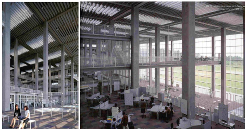
Figure 5. Suspended floors, Future University of Hakodate in Japan
