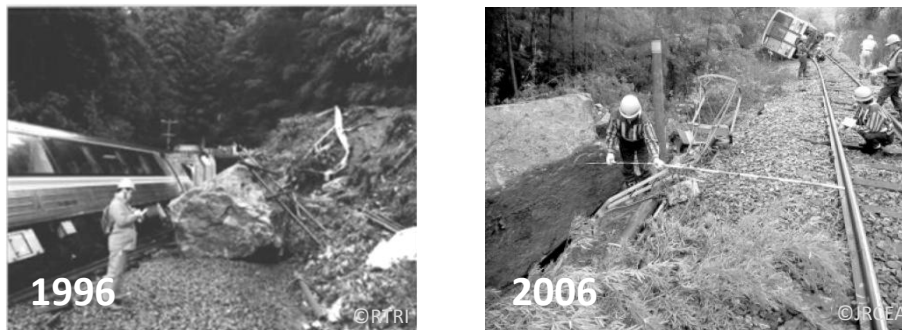
Figure 2. Examples of derailment damage by falling rock
