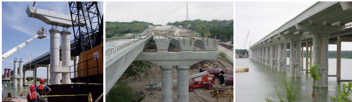
**Figure 2.1.** Lake Belton precast hammer head caps, Dacio Marin III, Texas DOT (2002)
