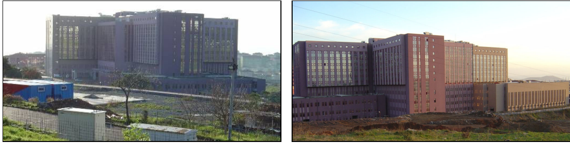
Figure 3. Existing condition of the hospital
