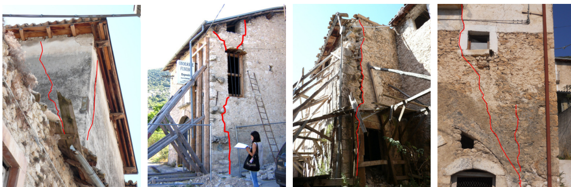
Figure 5. Damage mechanisms in San Pio delle Camere (buildings aggregates n° 352, 038, 134, 434 - see Fig.4).
