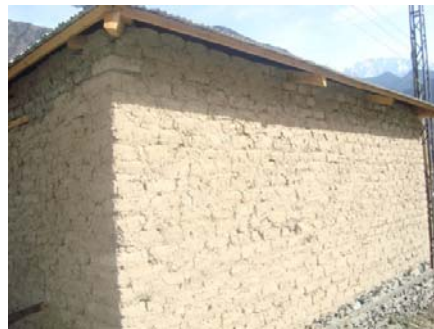
Figure 4.2. View of adobe house in Chitral
