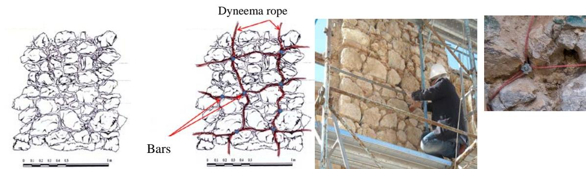
**Figure 2.5.** Panel n. 1 – Strengthening: the “Reticolatus” technique and bar detail.
