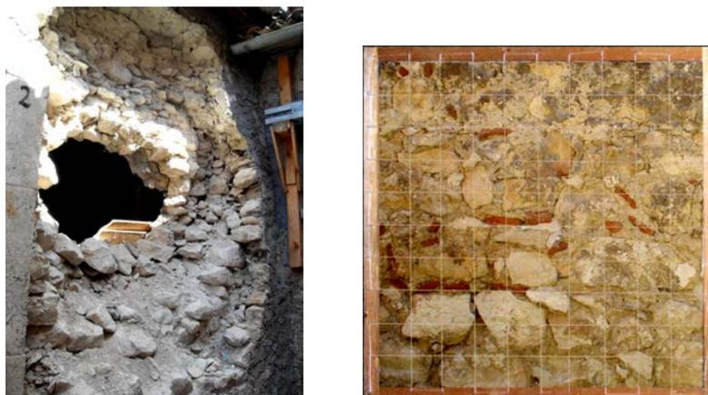
**Figure 6.6.** Masonry sampling – 1m x 1m – typology two, L'Aquila surrounding area. Local mechanism: out-of-plane – buckling occurrence.
