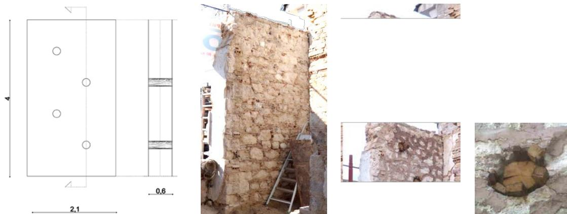
**Figure 2.10.** Panel n. 5 –Schematic plan for wooden headers setting and executive phases' photos. Wooden header and wedge-elements settled photo' detail.
