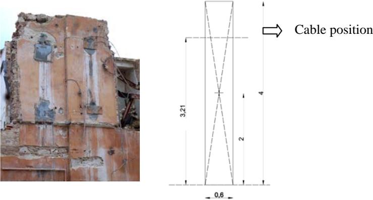
**Figure 3.1.** Panel n. 2 –Cable position and panel n.2 geometrical dimensions
