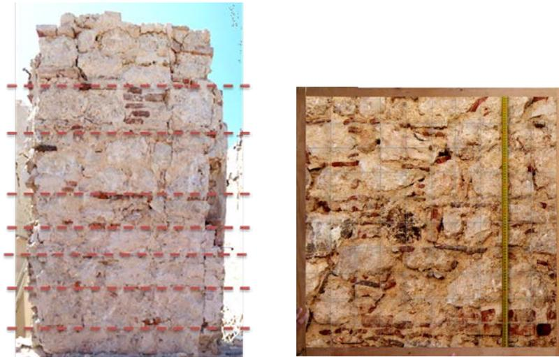
**Figure 5.5.** Masonry sampling (1m x 1m) typology one, L'Aquila historical centre. Local mechanism: out-of-plane - rigid block behaviour.
