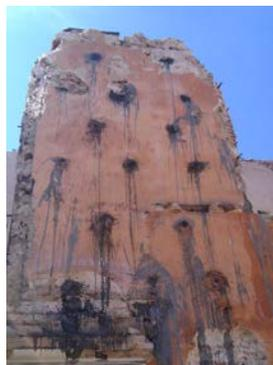
**Figure 2.2.** Panel n. 4 – Masonry reinforcing with anchors
