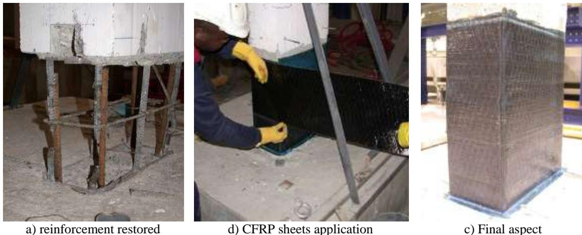
**Figure 1.3.** CFRP retrofitting
