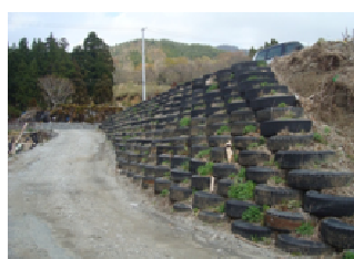
Figure 3. Tire retaining wall in Okirai (Photo taken after the compound disaster)
