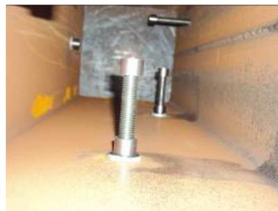
Figure 7. Blind bolts in a square hollow section
