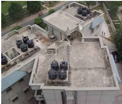
Figure 2.3. An existing building with acute plan irregularity
