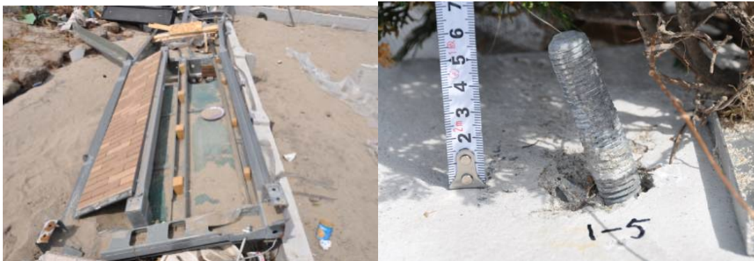
Figure 3. Deformed bolt and remained parts
