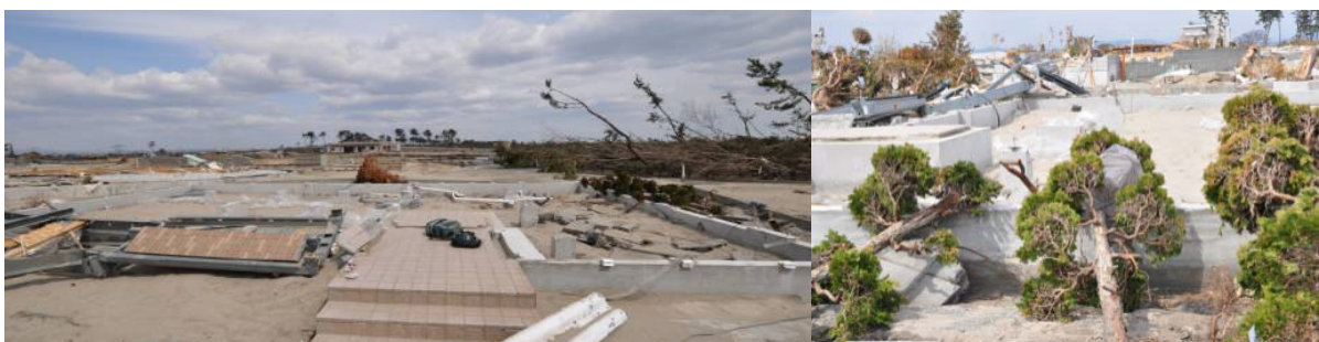
Figure 2. Foundation of the building after tsunami
