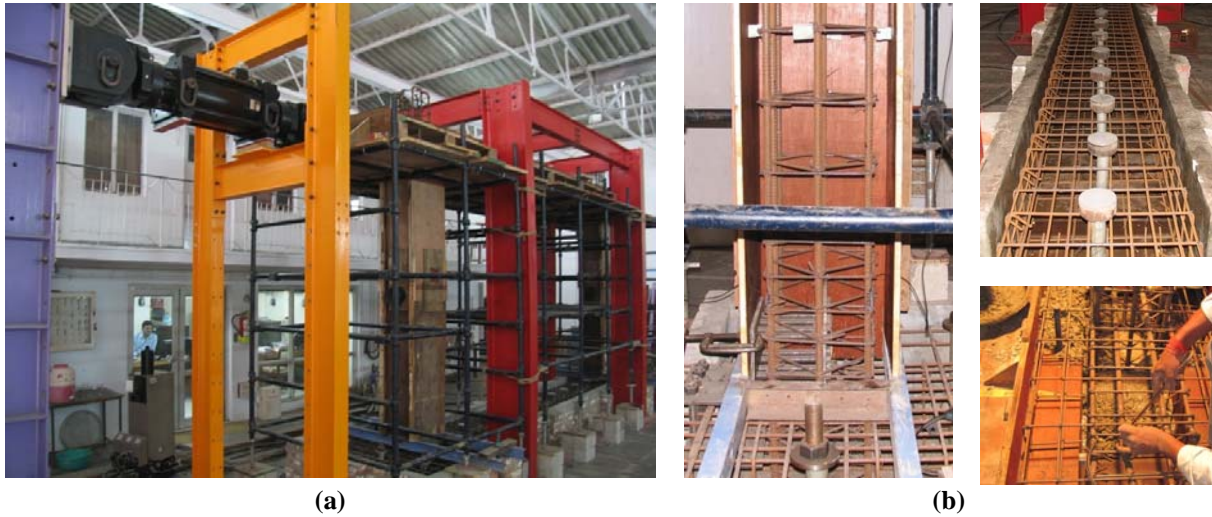
Figure 2.6 (a) Test frame during concreting showing reaction and lateral support frames, (b) Reinforcement details of column (left), footing (top) and beam (bottom)
