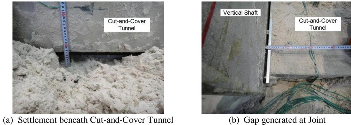
**Figure 10.** Damage Condition of Joint between Vertical Shaft and Cut-and-Cover Tunnel
