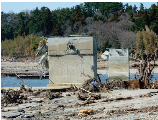
Figure 1. Damage to steel pipe with 2400mm diameter (Miyagi Pref.). ( http://www.pref.miyagi.jp/kigyo/ )
