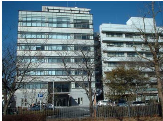
Figure 2.1. External view of the BRI annex building
