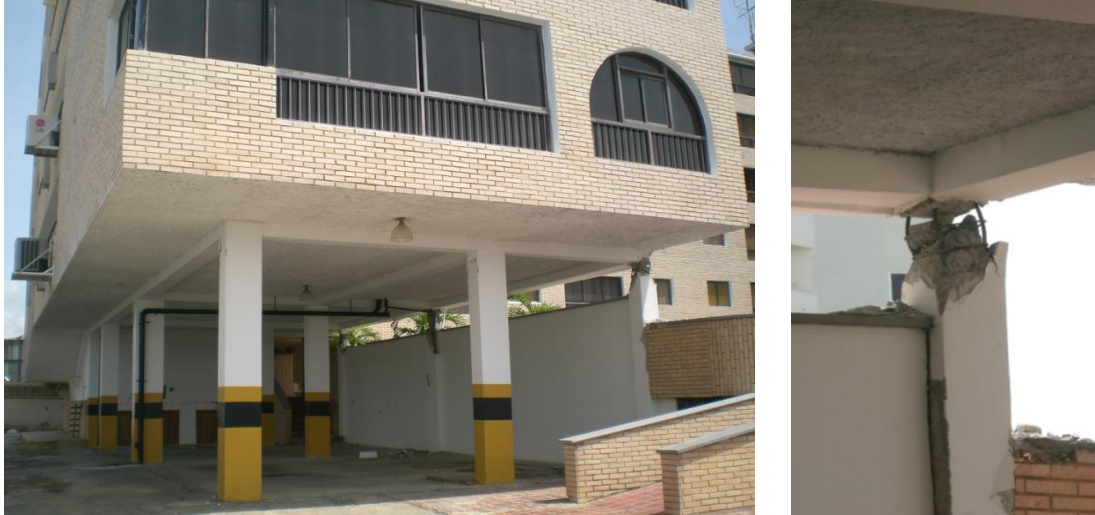
Figure 8: Free story and short column effect
