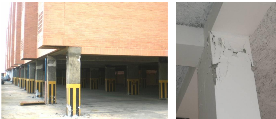
Figure 7: Typical soft story mechanism at free story
