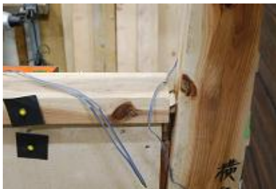
Figure 10. Joint of window sill-column at a drift of 6.6% (2W b )
