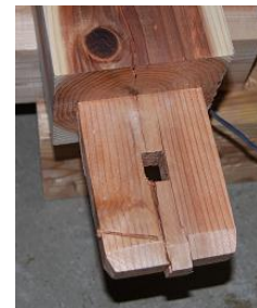
Figure 12. Shear failure of tenon (2HW b )
