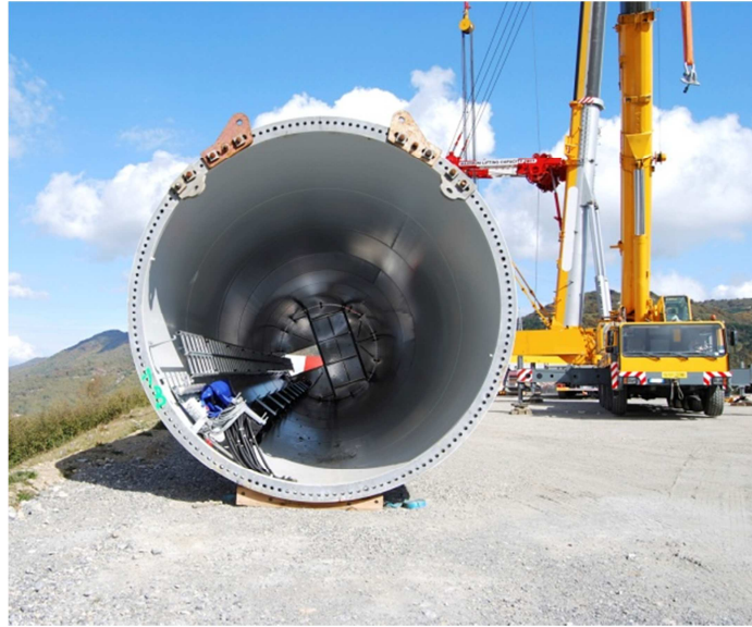
Figure 4. Example of cross-section of a wind turbine tower shows high slenderness ratio.
