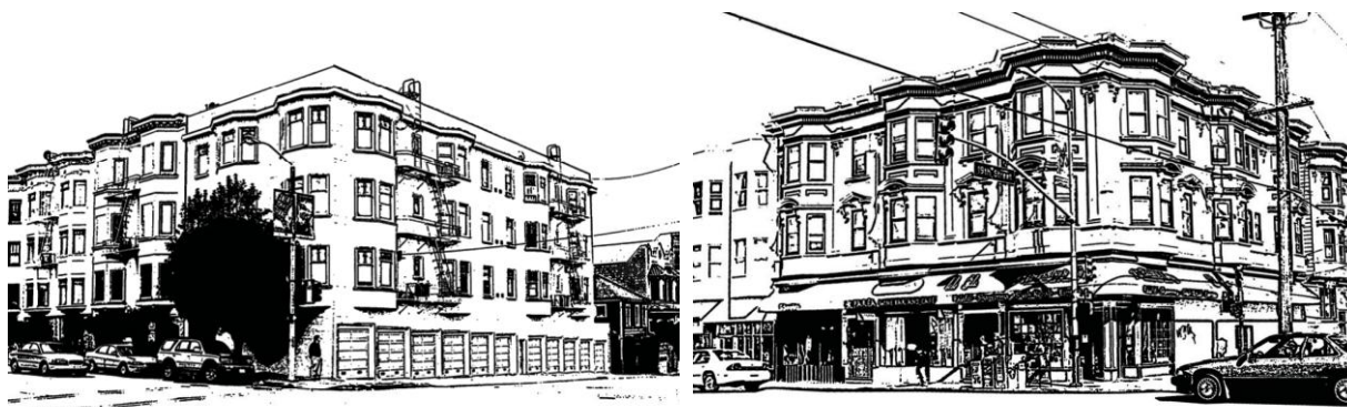
Figure 3. Images of two multi-unit, wood-frame buildings that may have soft-stories
