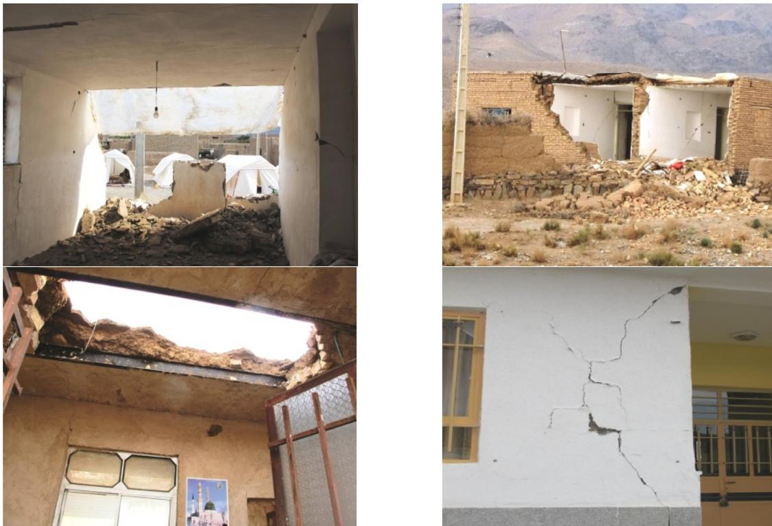
**Figure 3.** Field photographs (a) Typical adobe-brick house at Kelu (b) Collapse started in the corner where it was easier to initiate instability. (c) Collapse of masonry arches due to the movement of the roof (d) Partly damage of the reinforced concrete elementary school building
